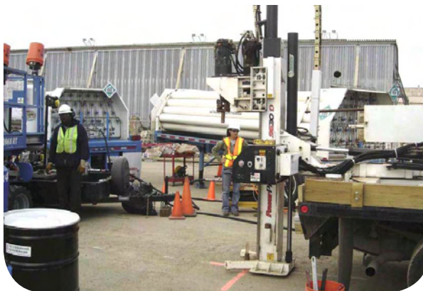
Pneumatic fracturing at the Hunters Point Naval Shipyard Superfund site
