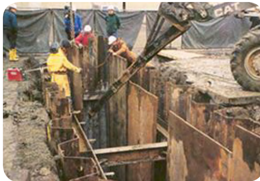
Construction of a PRB in Sunnyvale, CA
