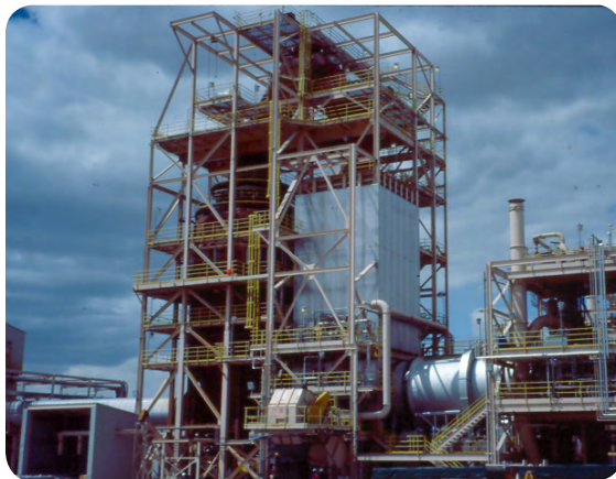
Example of offsite incinerator.
