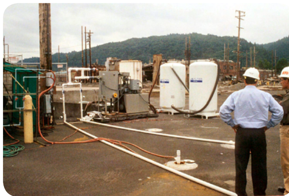
Above-ground treatment system includes two tanks of activated carbon.
