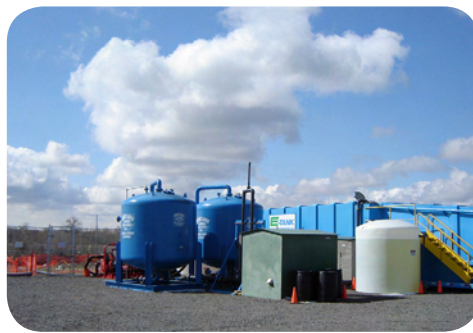
Outdoor Treatment Facility
