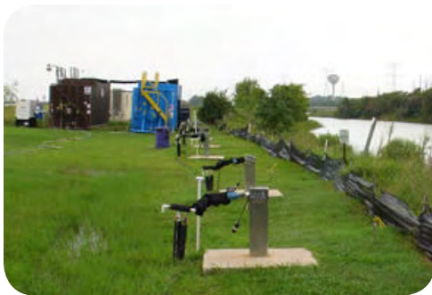
Groundwater Pumping Wells
