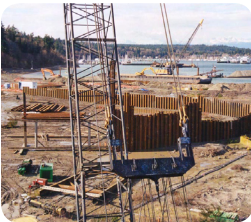
Installation of sheet piling
