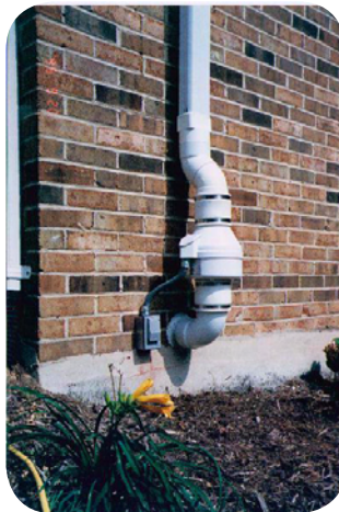
Typical fan and vent pipe.
