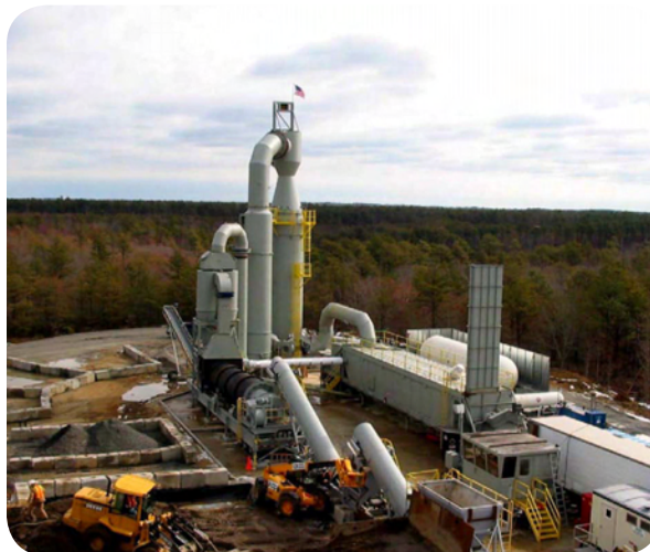
Onsite thermal desorber.
