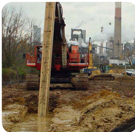
Excavation of a slurry wall trench
