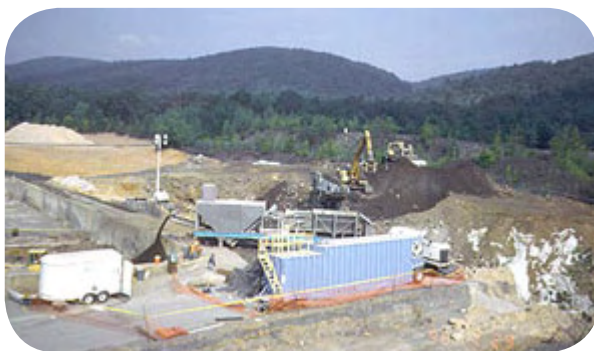
Contaminated soil mixed with cement in a pug mill is spread on the ground as pavement.
