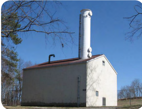
Air stripper and treatment building
