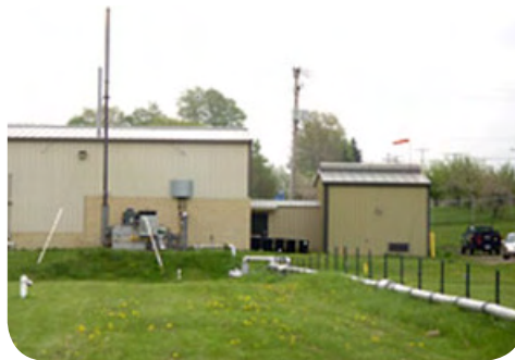
Groundwater Treatment Building
